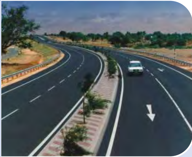
Sira Bypass in Karnataka was built in 2002 and forms a network with the ever-busy National Highway 4
