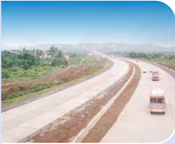
Mumbai-Pune Expressway, the most premier access-controlled highway in the country, was built using latest equipment such as slip-form pavers and auto-controlled batching plant. This world-class road has drastically reduced the travel time between the two cities.
