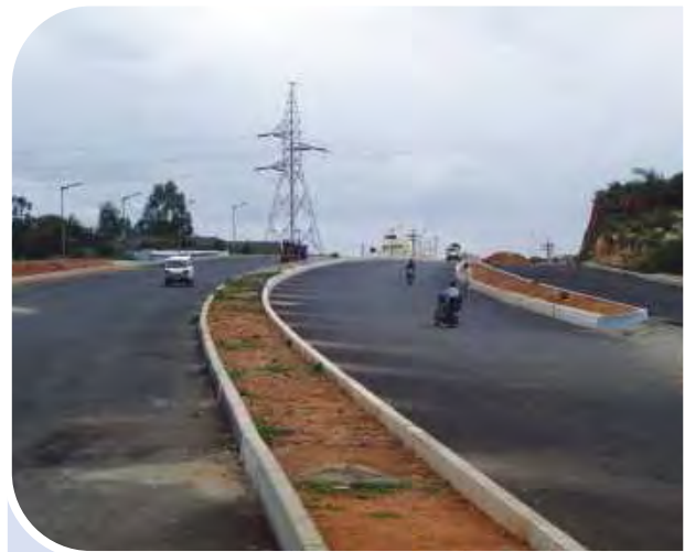
The BDA Outer Ring Road project is built along 5kms to decongest the core part of the Bangalore.
