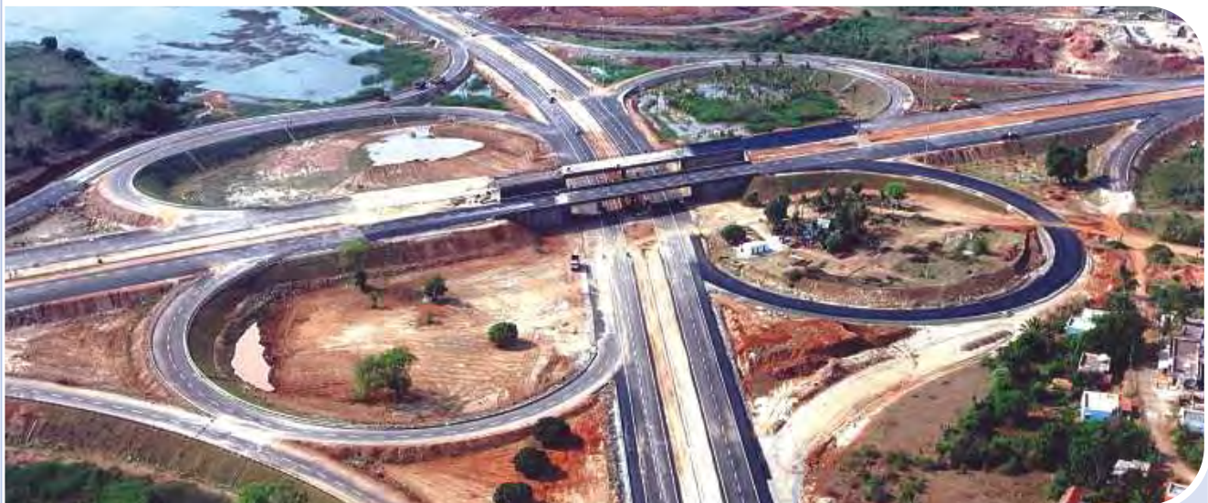
NICE Project is one of the most formidable projects being executed by Maytas Infra. The project includes 2-km expressway and a major clover-leaf interchange for uninterrupted flow of traffic
