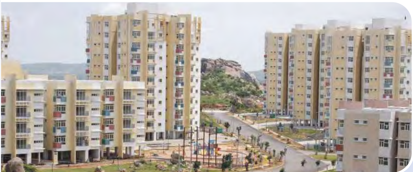
Singapore Class Township built in 2005 offers a built-up area of about 28,00,000 sqft at Pocharam near Hyderabad
