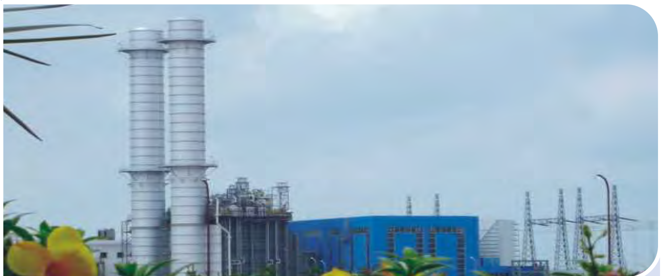
Gautami Power Project located in East Godavari district is a 460 MW gas based power project
