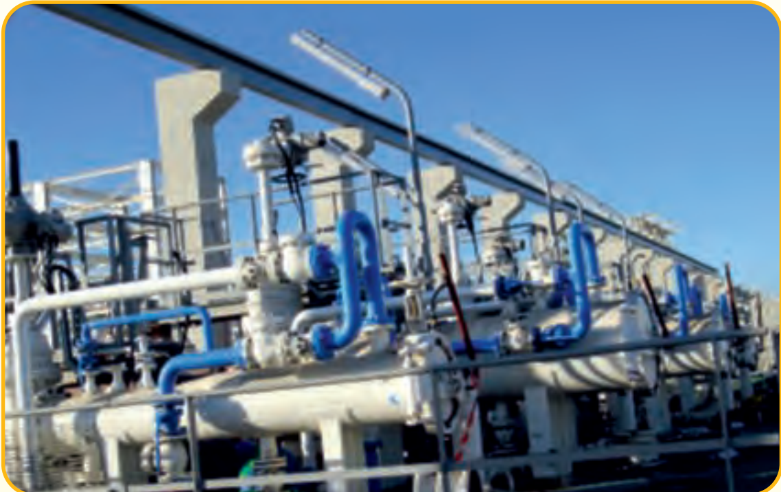
Pig Launcher & Receiver - Fujairah Jettyline Works
