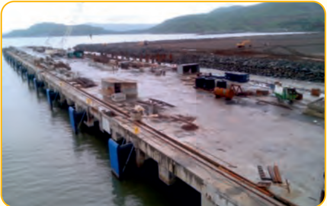
Berth No.4 Front View - Dighi Port, Raigadh, Maharashtra
