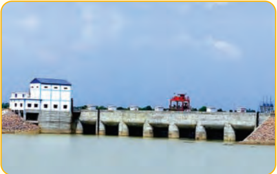
Anuppur Barrage Project at Son River, Anuppur District, Madhya Pradesh
