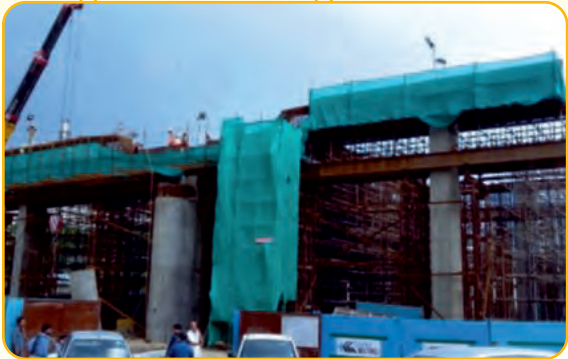
Rapid Metro Rail Gurgaon (RMRG) Phase-II Station Building - Construction in progress
