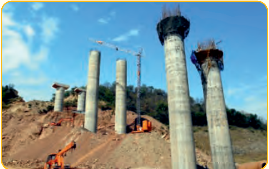
Sub structure work in progress at Km 26.184 Major Bridge at Kiratpur – Ner Chowk Road Project, Himachal Pradesh
