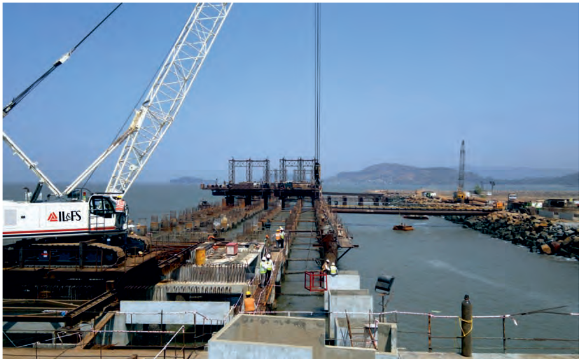
Precast Erection in Progress at Dighi Port, Raigadh, Maharashtra
