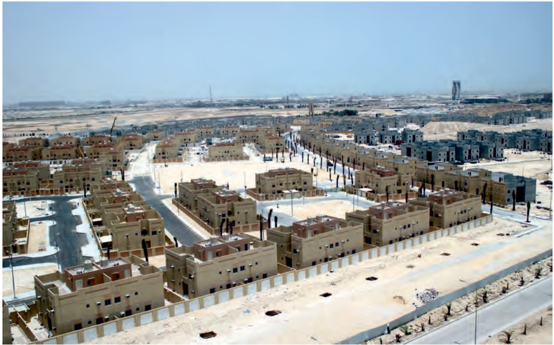
National Guard Villas at Saudi Arabia National Guard Housing Project (SANG), Dammam, KSA
