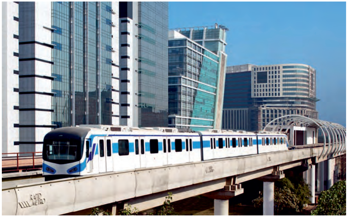
Rapid Metro Rail Viaduct, Gurgaon
