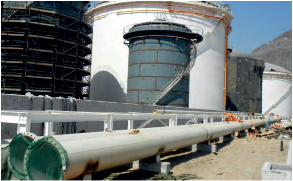
Tie in Point with Jettylines (Fujairah Jettyline Works)
