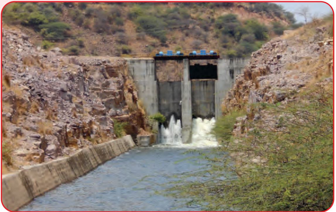
Chitravathi Balancing Reservoir Right (Lingala) Canal, Kadapa District, Andhra Pradesh
