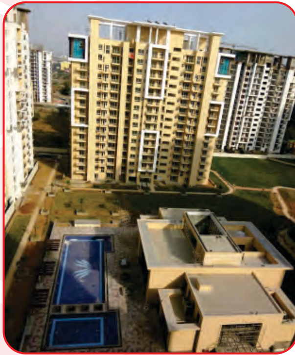
Palm Garden Residential Project, Gurgaon, Haryana
