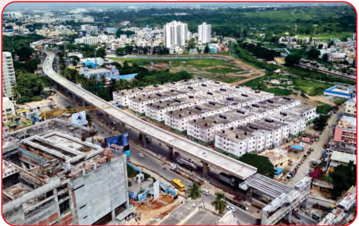
Bangalore Metro Rail Project, Phase-2, Bengaluru, Karnataka
