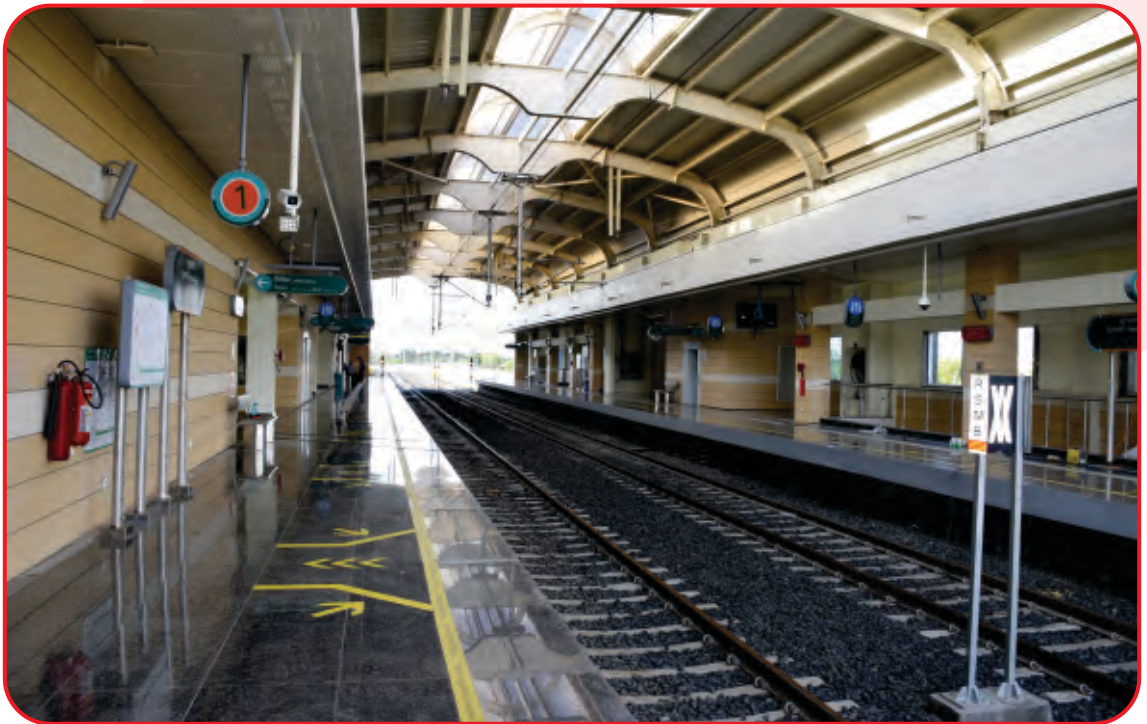
Nagpur Metro Rail Project, Nagpur, Maharashtra
