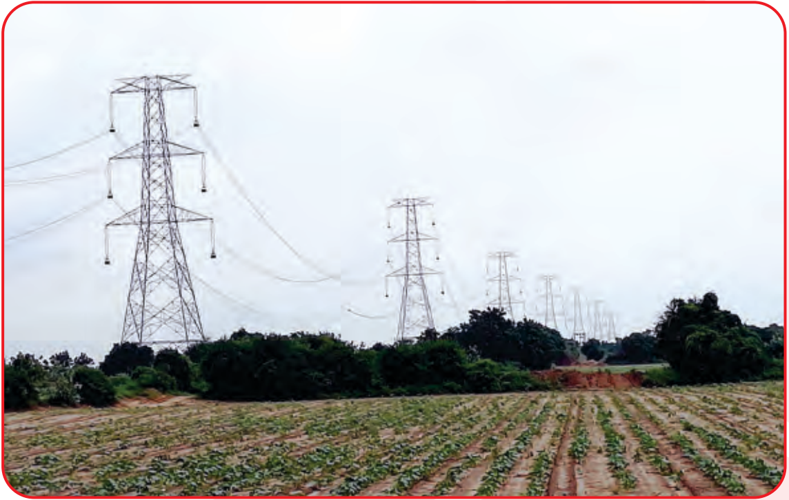
765kV D/C Bhuj-Banaskanta Turnkey Transmission Line Project, Gujarat
