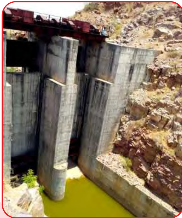
Lingala Canal Project, Kadapa District, Andhra Pradesh
