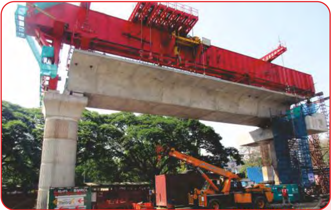
Bangalore Metro Rail Project, Bengaluru, Karnataka
