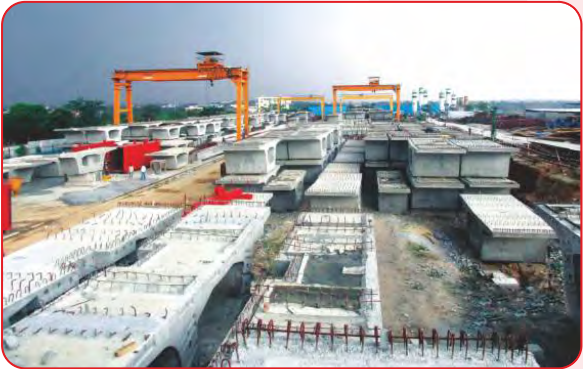
Bangalore Metro Rail Project, Bengaluru, Karnataka
