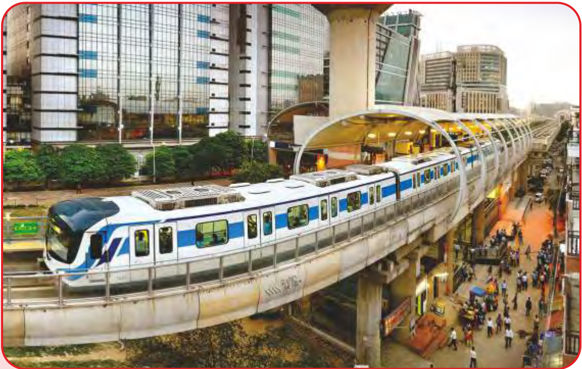
Rapid MetroRail Gurgaon Project, Gurgaon, Haryana
