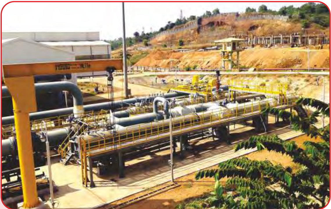
Mangalore Port to Mangalore-Padur Pipeline Laying Project, Karnataka
