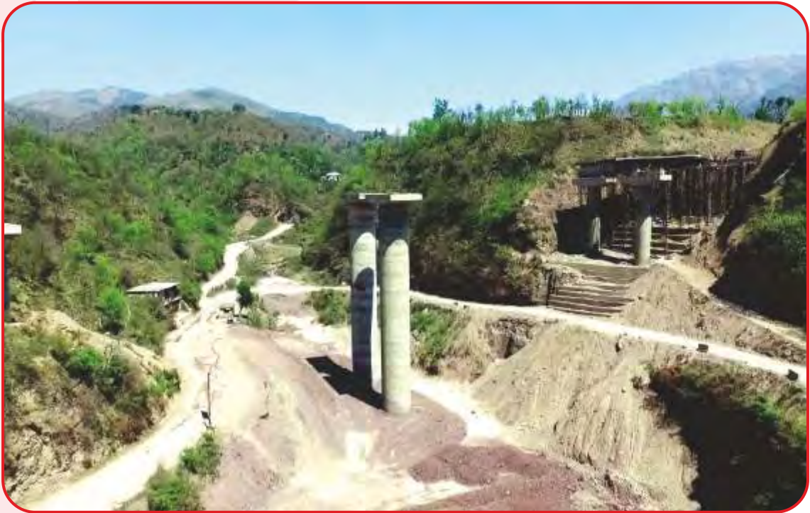
Four Laning of Kiratpur Ner Chowk Section of NH-21, Himachal Pradesh
