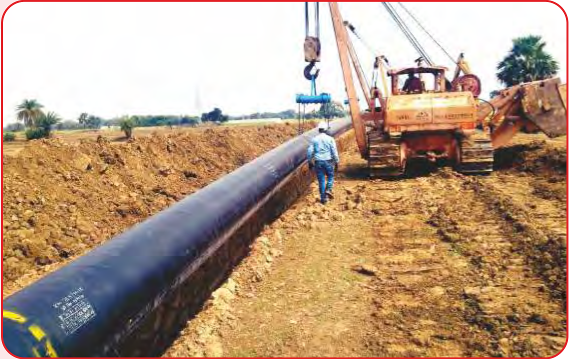
Phulpur-Haldia Pipeline Project Lowering at Chainage 313, Bihar
