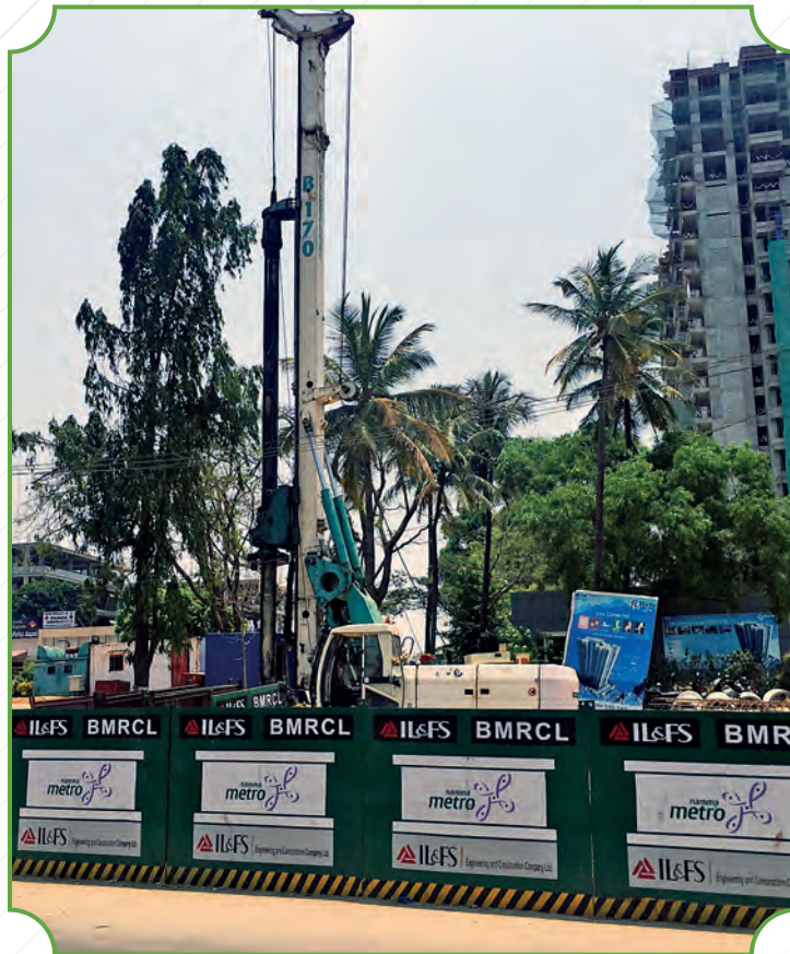
Work in progress at Bangalore Metro Rail Project, Karnataka
