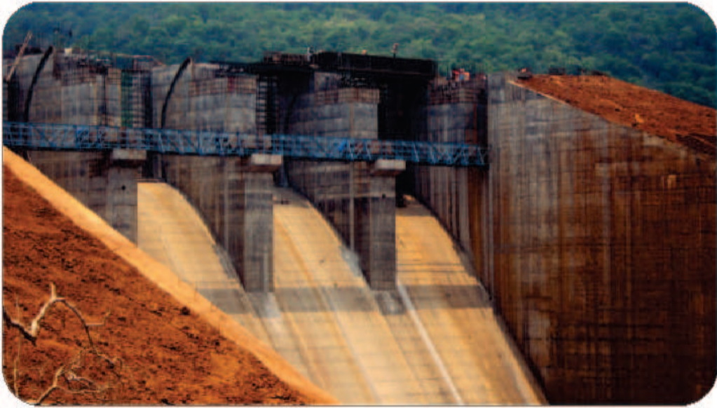
Bhupathipalem Reservoir Project, Andhra Pradesh
