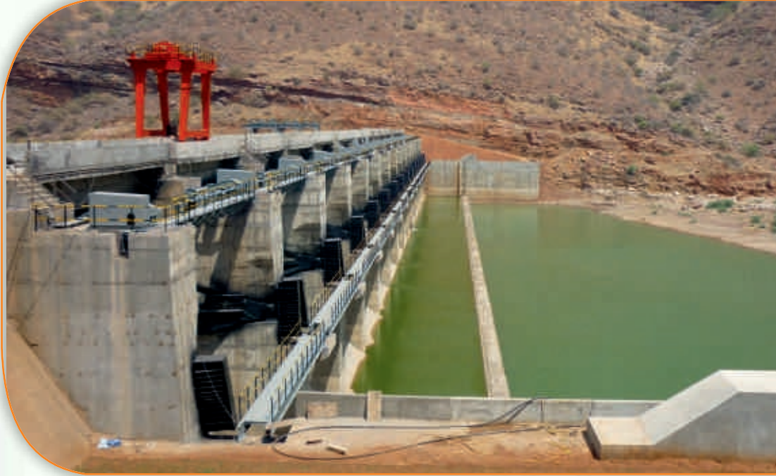
Galeru Nagari Sujala Sravanthi (GNSS) Project, Kadapa, Andhra Pradesh
